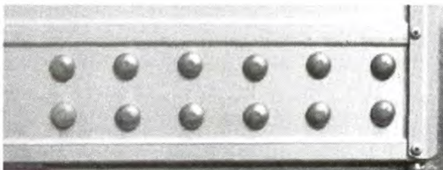
Figure Typical Huck Bolt
